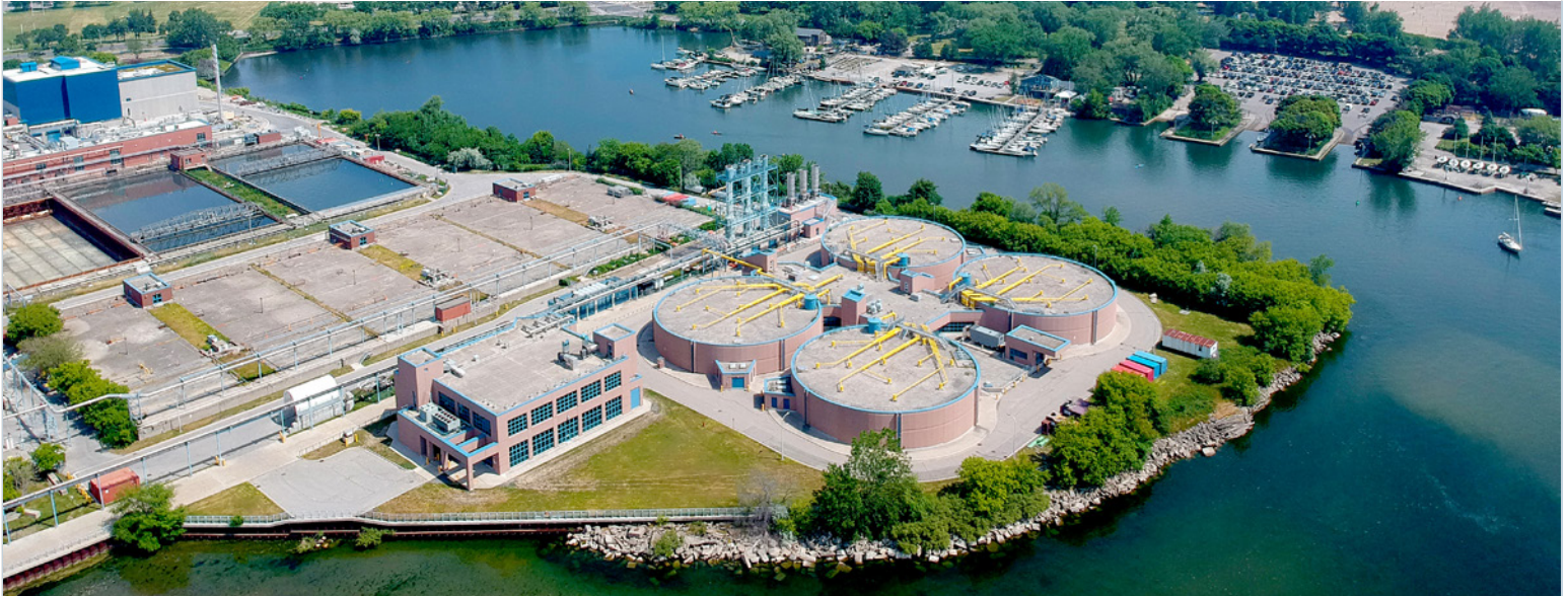
Ashbridges Bay Wastewater Treatment Plant, Ontario.
