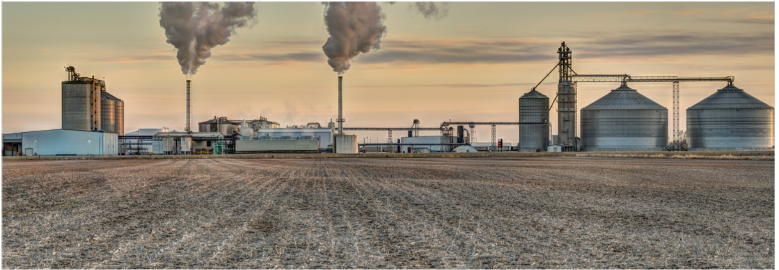
Ethanol Plant. Adobe Stock
